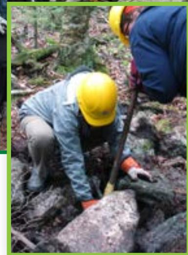
place flat rocks in them for proper footing. Big rocks were split into smaller rocks to fill in areas around the holes. Then the final touch: gravel to smooth out and cement the rocks in place. Team members took turns to carry loose shale in buckets up the trail while a few used hammers to split the rocks.
